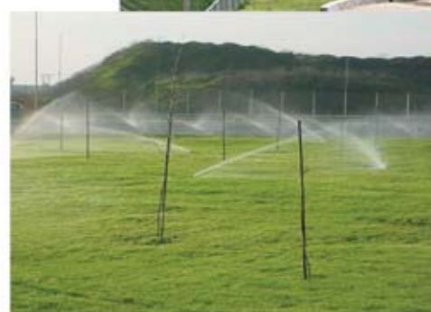
With vandalism to irrigation components eliminated, Santiago's highway landscaping stays lush and green.
