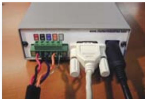
Figure 9: CCC GCBL wiring
