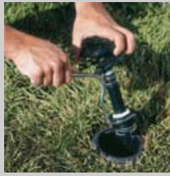
1. Remove internal assembly of existing sprinkler.
