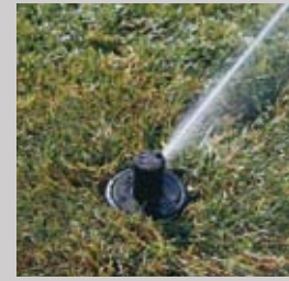
3. Set watering pattern to desired arc.
