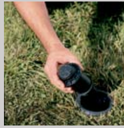
2. Thread entire ATR body/riser into canister.
