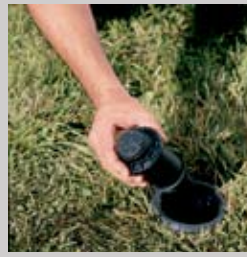
2. Thread entire ATR body/riser into canister.
