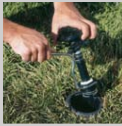
1. Remove internal assembly of existing sprinkler.
