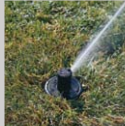
4. Set watering pattern to desired arc.
